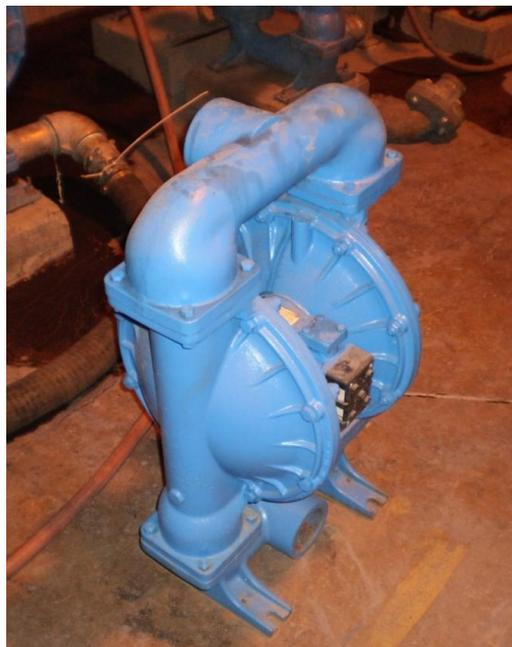
*Figure 2. Air pumps use seven times more electricity than electrical pumps*
